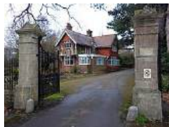
Lodge, gates and railings
