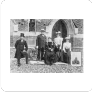
Henry Ward and John Lambert Walker during construction
