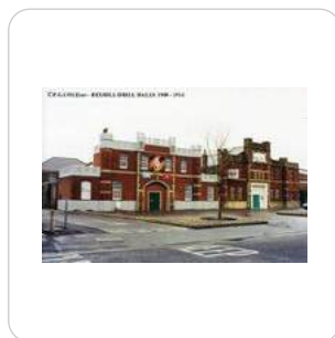
Showing existing and demolished Drill Halls
