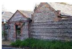
Garden House garage and walls
